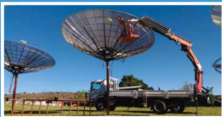
These are some of the six-metre wide HIRAX prototype radio dishes installed at the Hartebeesthoek Radio Astronomy Observatory.
